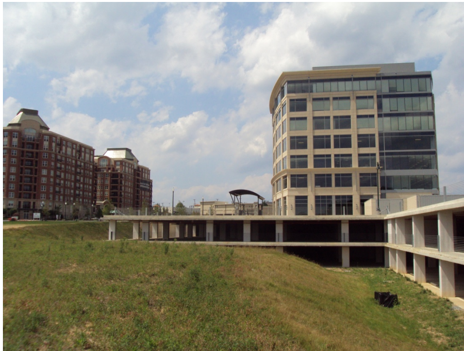
Figure 6: View from North
